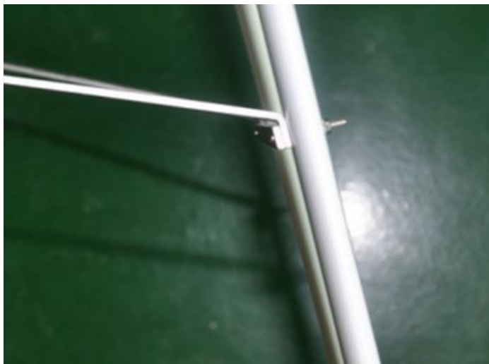
Fix it up to aluminium sheet with screw as shown
